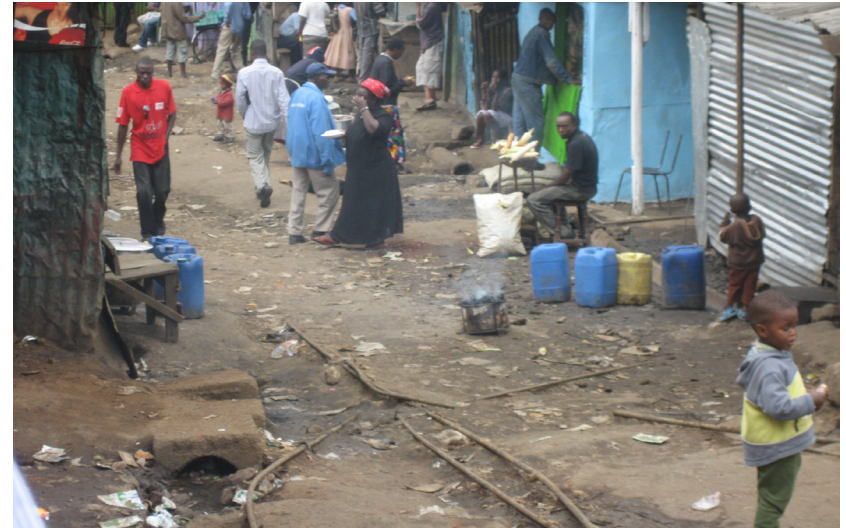
Above: random exposed water pipes, frequently contaminated by sewage Left: typical yard tap
